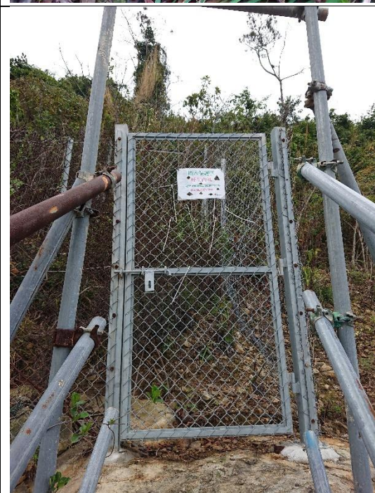
Photo 2 – Current situation of fencing and warning sign
